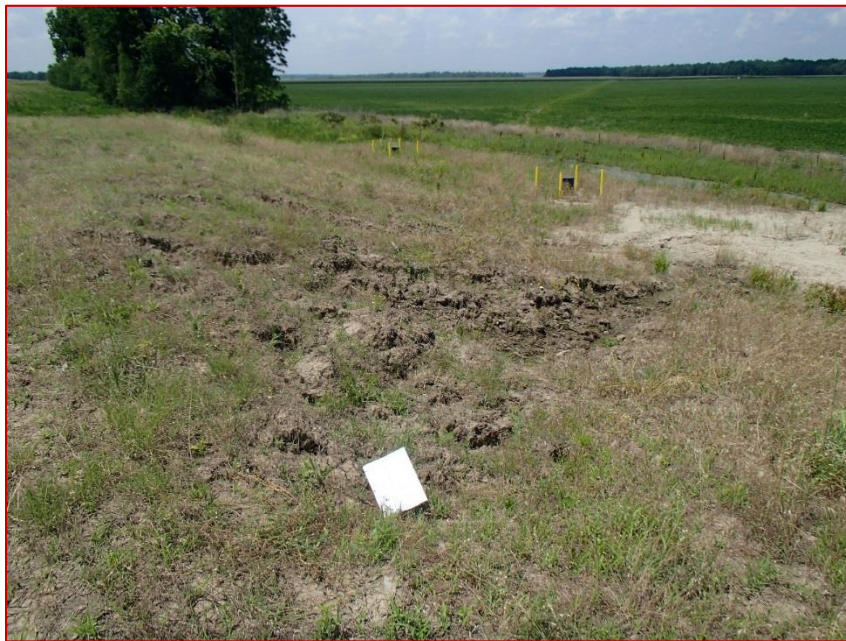
Figure 1.5 Relief wells installed on the landside of the levee at Francis, MS.
