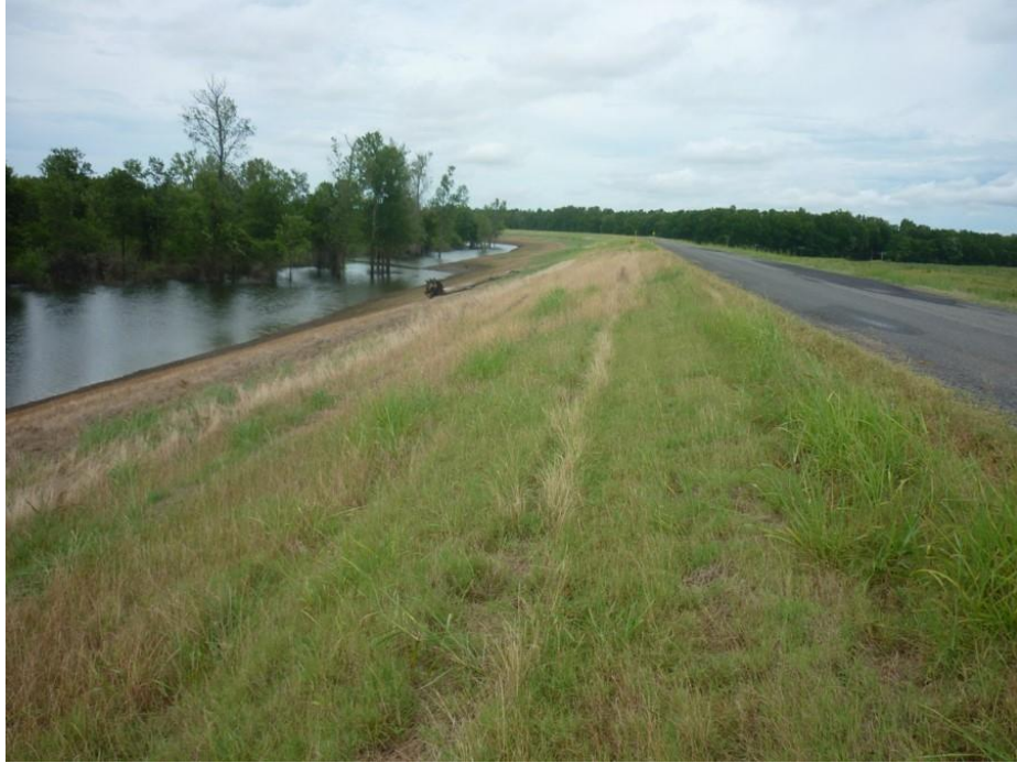
Figure 1.1 Earthen Levee on the banks of Albemarle Lake, MS, a Mississippi River oxbow.
